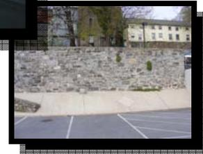
PCI evaluated the condition of an existing wall separating two levels of a parking lot. The existing wall was not designed to be a retaining wall and was failing. The result of the investigation lead to the design of a one hundred seven feet long stand alone steel reinforced concrete retaining wall to support the upper level parking and travel lane. The project included site work for grading and new asphalt paving, guardrail and protective fencing.
